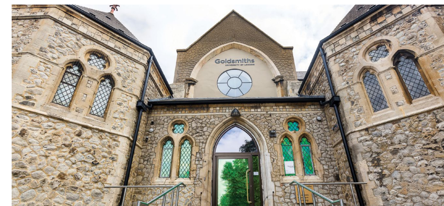
The exterior of St James Hatcham after renovation
